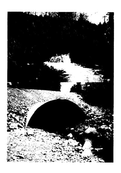
The Brickyard Road crossing over Bear Creek was replaced with a large, fish-friendly culvert, an improved road and a steel guardrail. Tillamook County Public works took on all project management and contract management duties and oversaw the project to a successful completion, on time and on budget.
