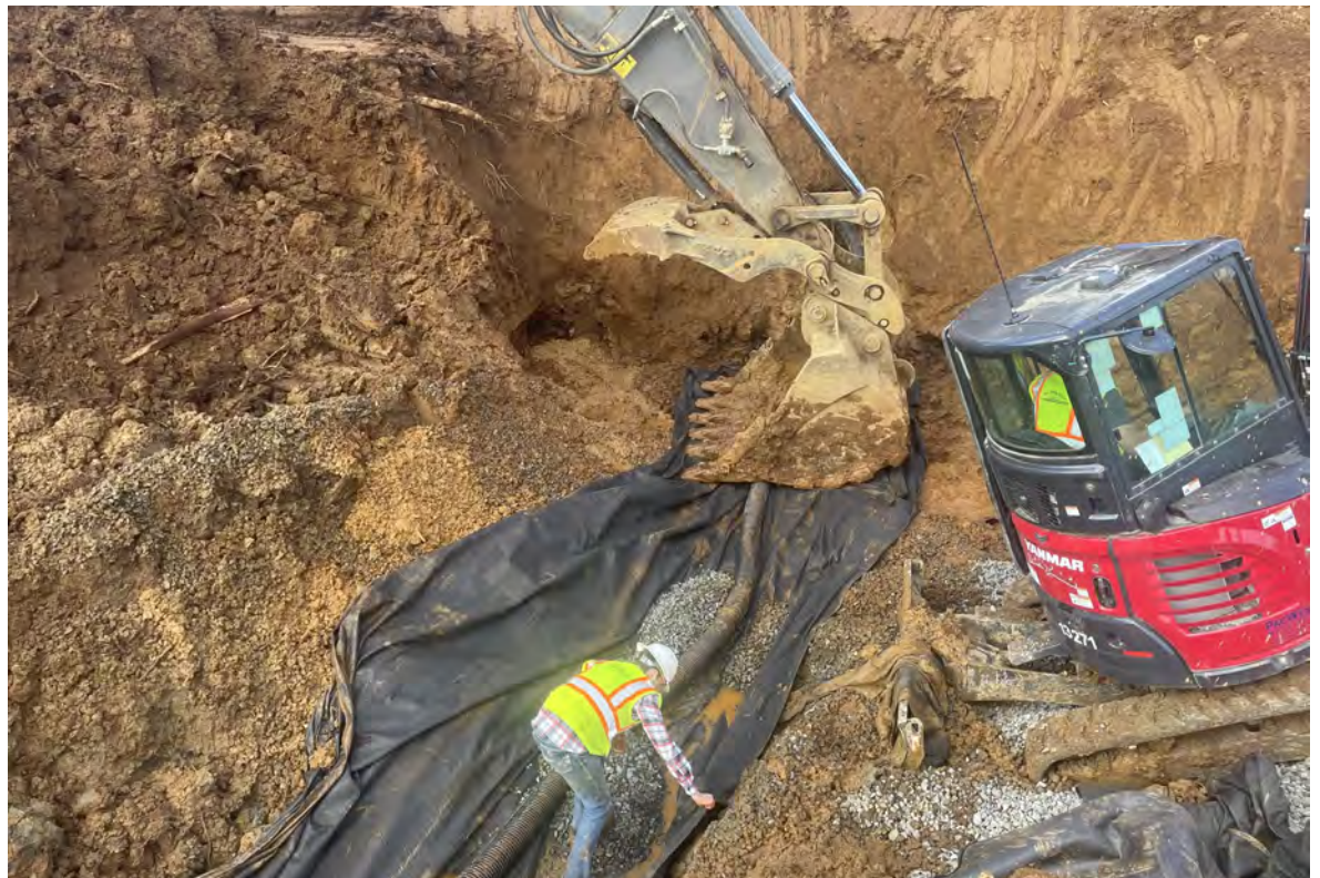
View of subsurface drain installation beneath MSE Wall No. 3 on 03/29/23.
