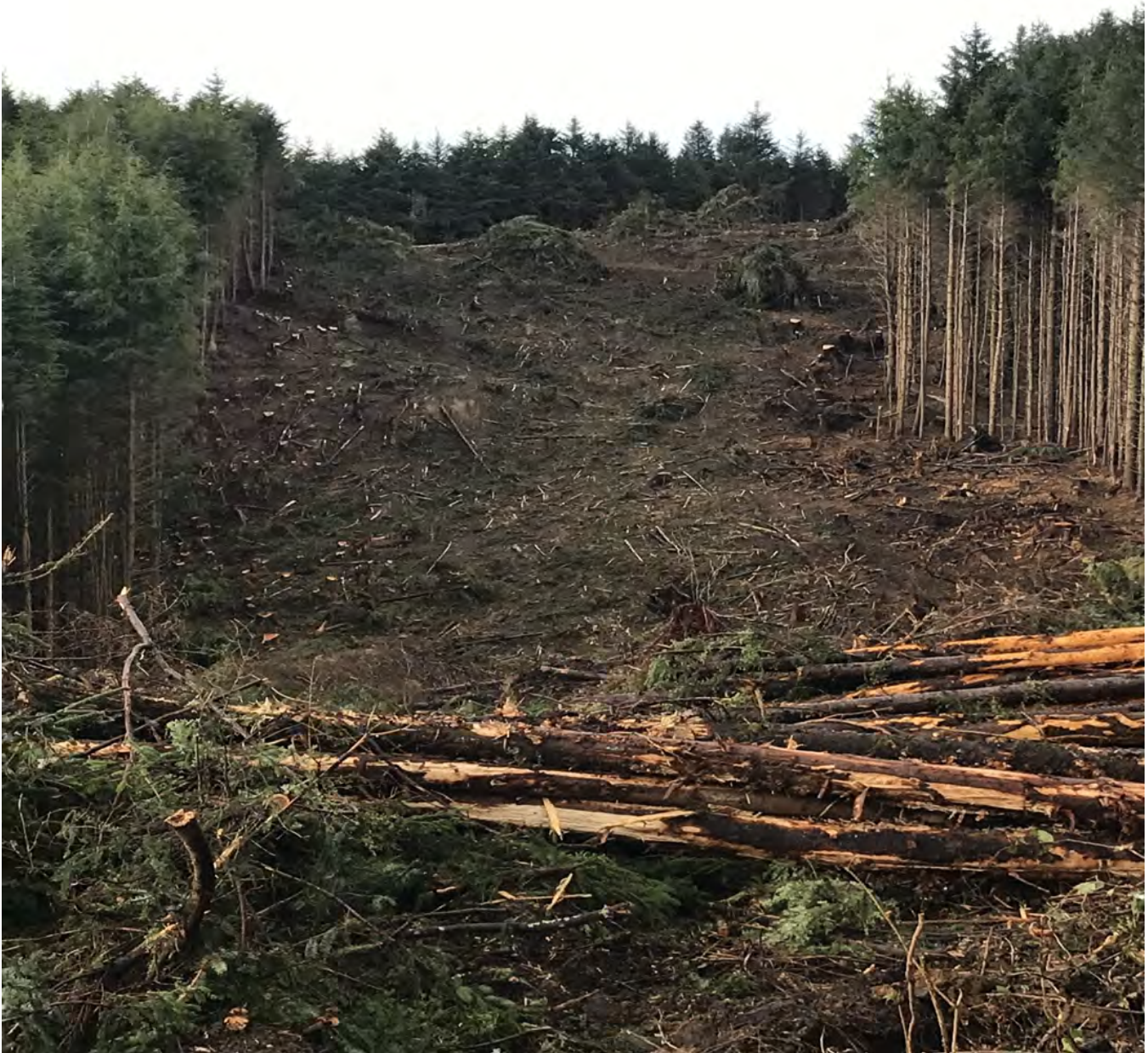
Station 333 slope after timber has been processed.
