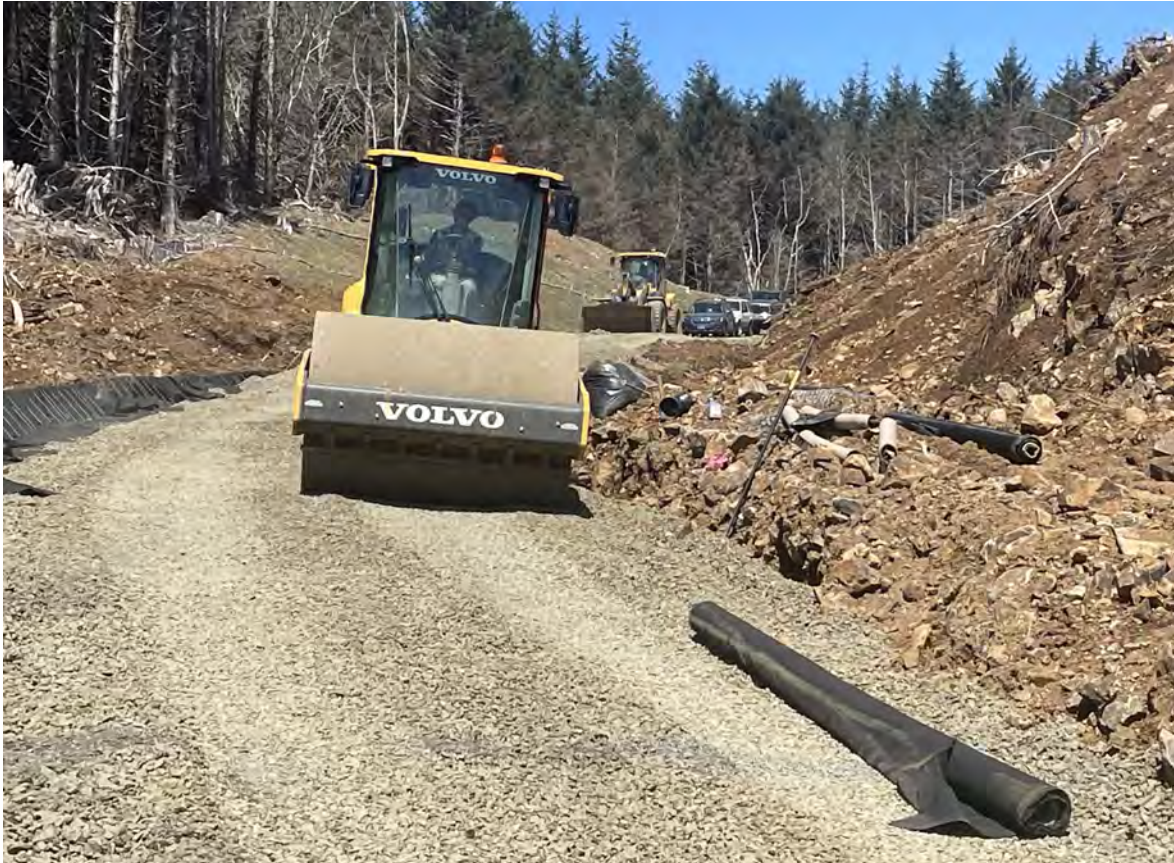
View of consolidation of MSE Wall backfill material.
