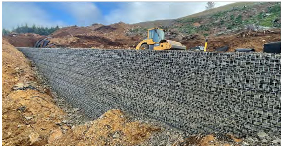
View of MSE Wall No. 3 after the completion of 11 courses.
