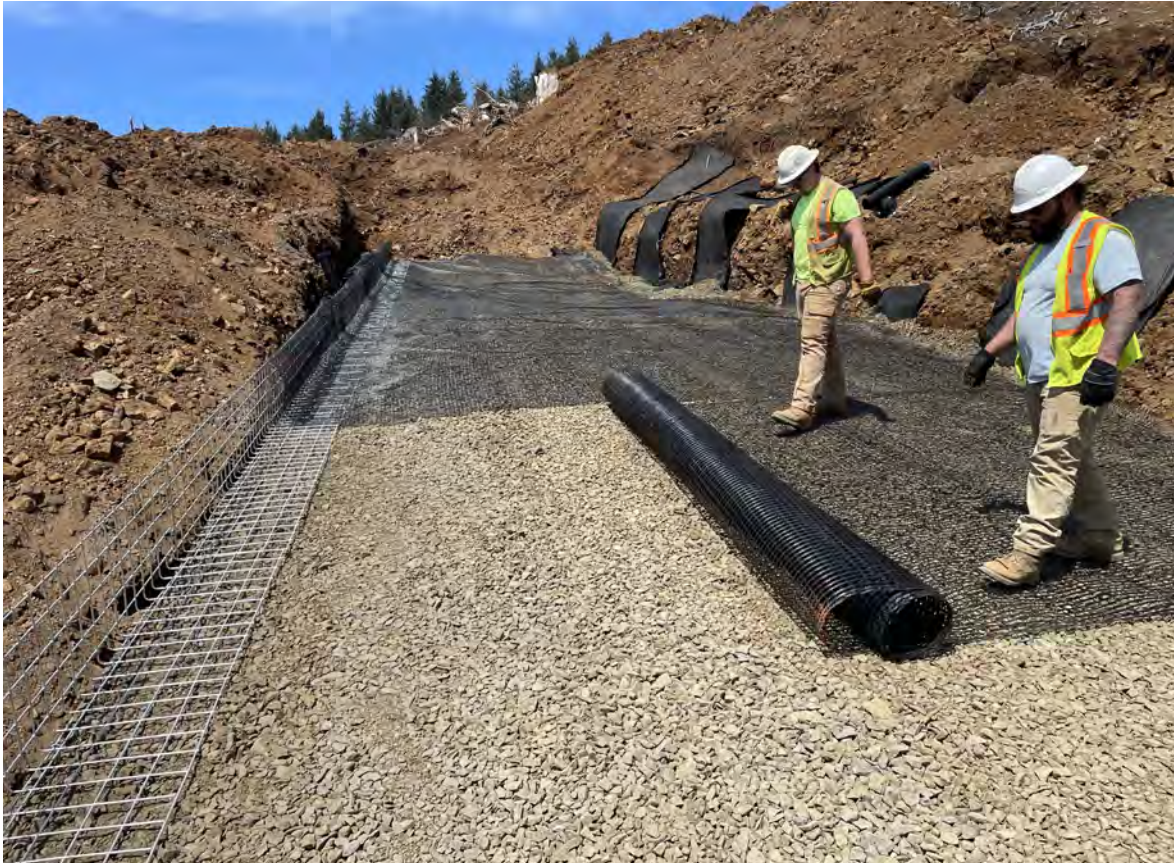
View of MSE wall geogrid reinforcement being placed on.
