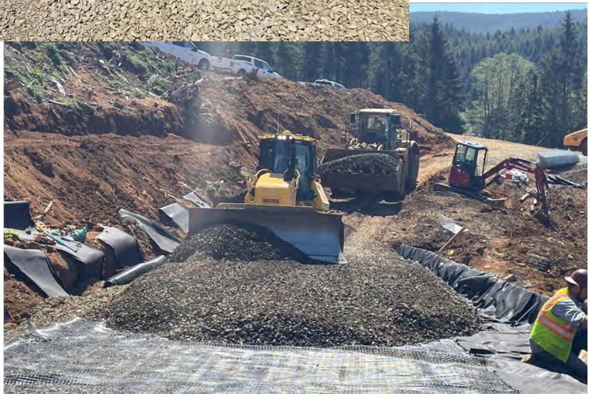
View of MSE wall structural backfill placement.
