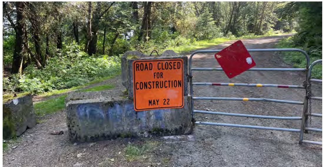
View of lighthouse gate showing newly installed sign informing the public of road closure of old Cape Meares Loop. Western Federal Lands Highway Division
