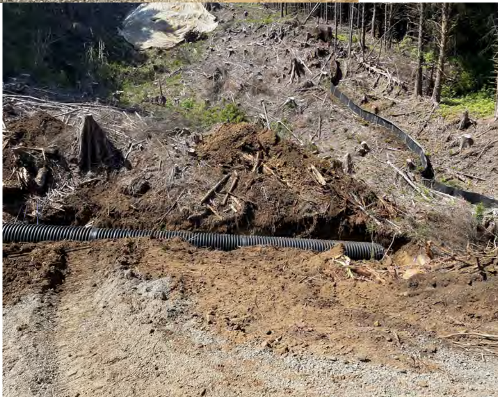
View of MSE Wall No. 1 36" culvert at stream 4.
