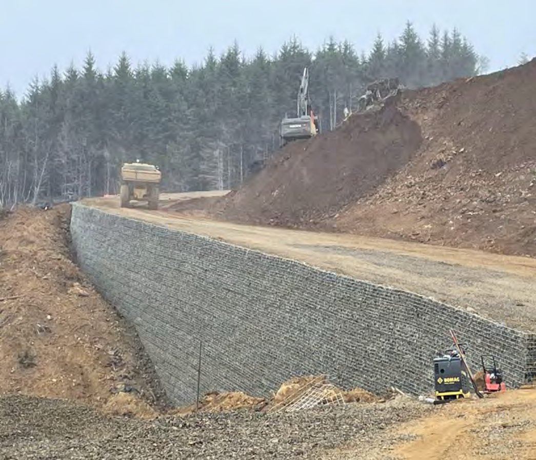
View of Lt side cut slope work above MSE Walls 2 & 3.
