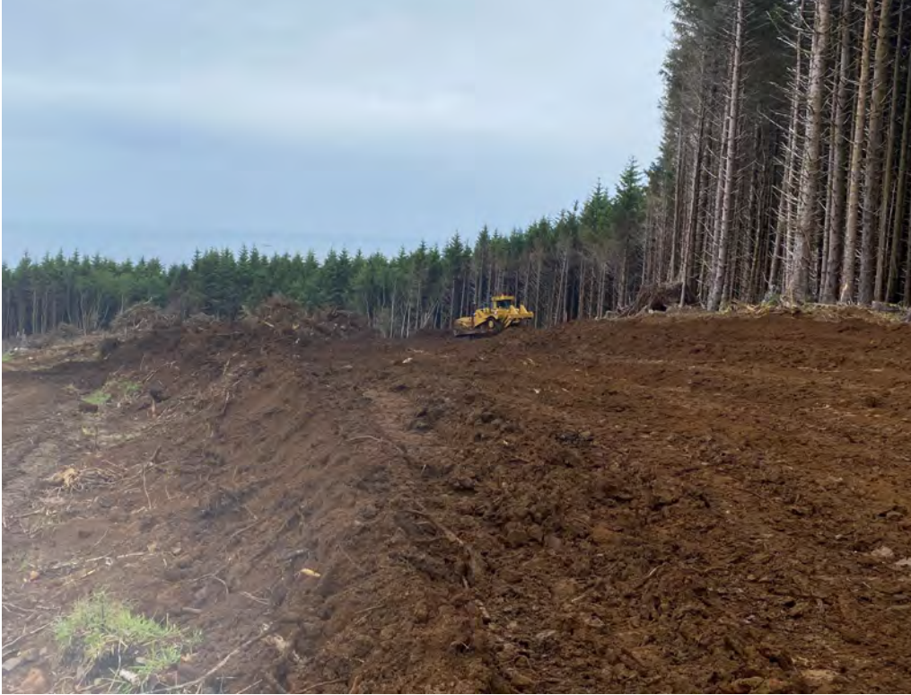
Dozer conserving material
