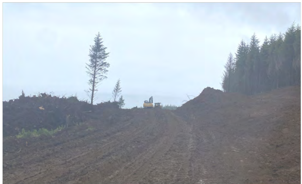
Excavator pulling stumps/ piling slashes
