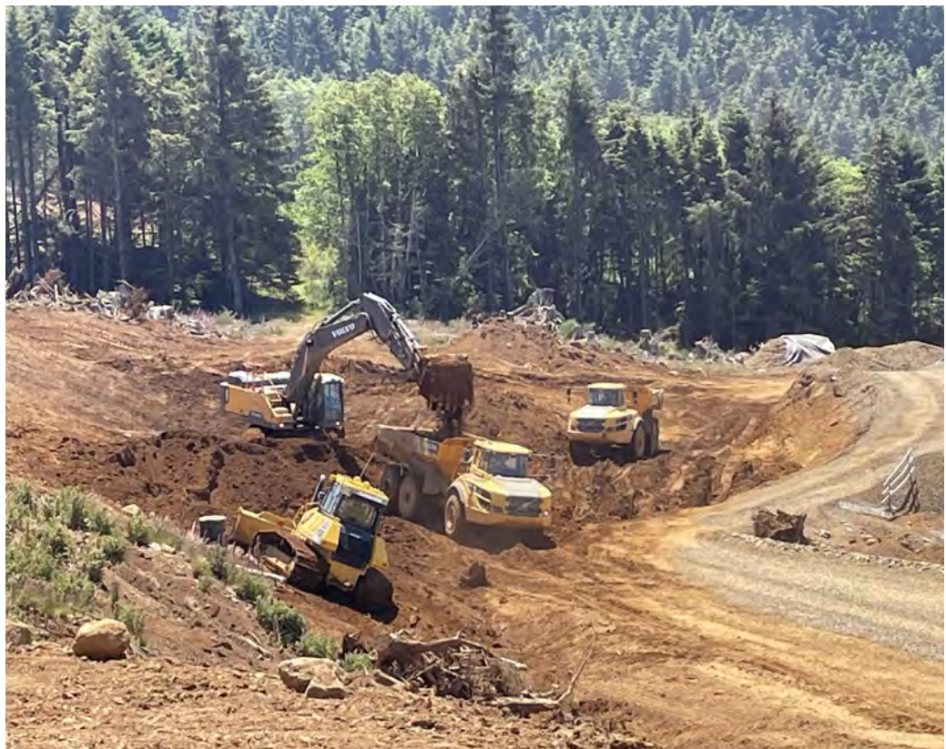
View of roadway excavation near the south entrance of the project.
