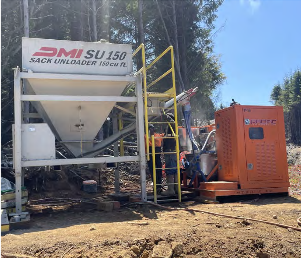
View of onsite grout production before being pumped into ground anchors.
