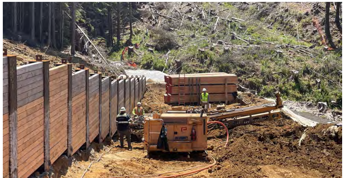
View of horizontal drilling at soldier pile wall during ground anchor installation.
