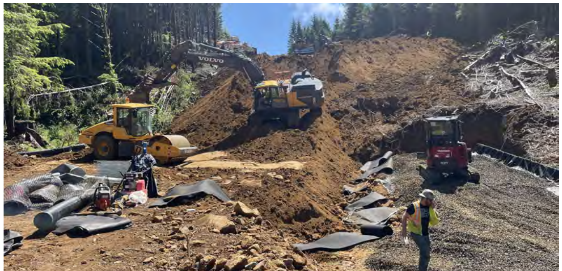
View of roadway fill operations behind MSE Wall.
