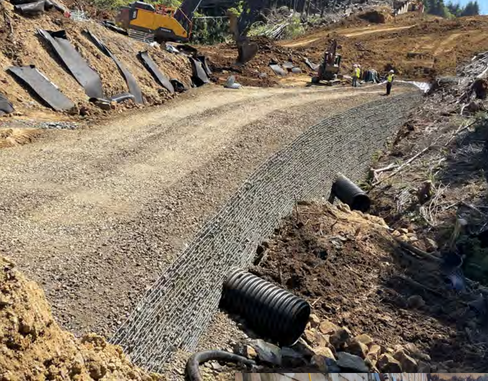
View of MSE wall construction progress.
