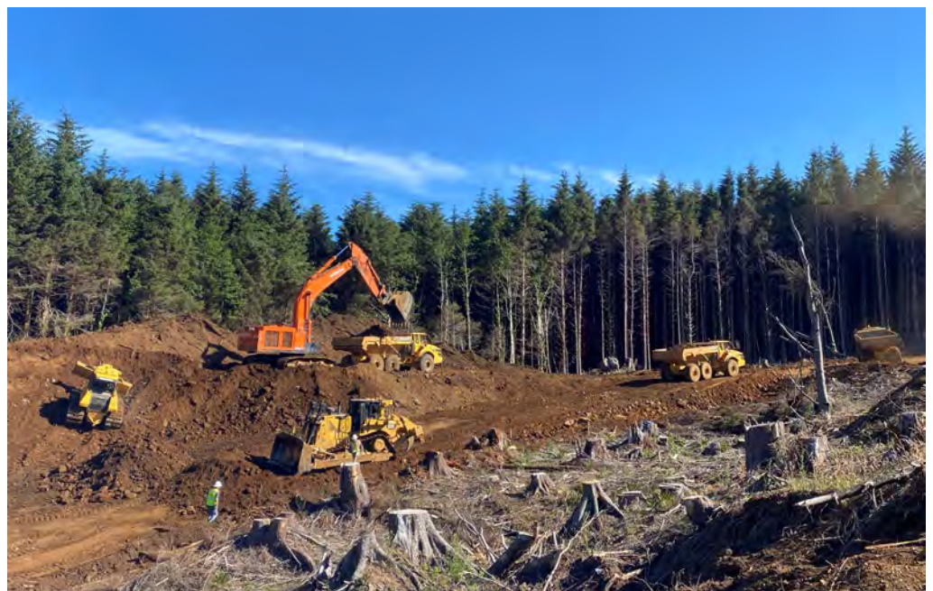
Excavation at st370.
