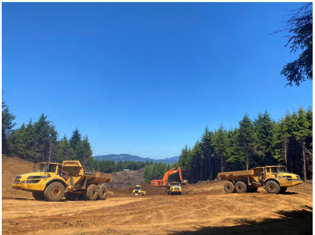
Excavation at st330.
