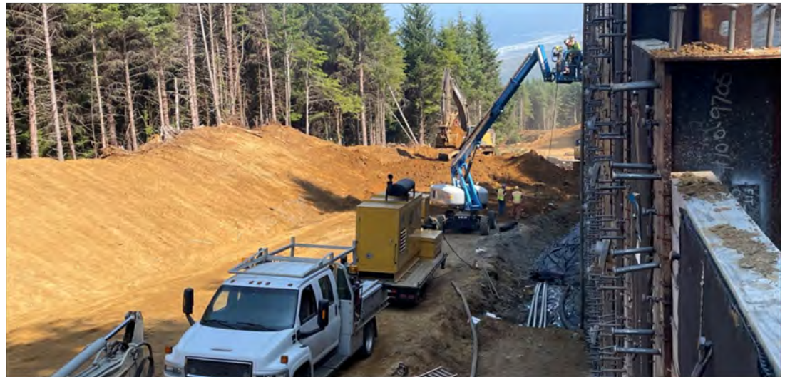
View of headed shear stud welding at the soldier pile wall.
