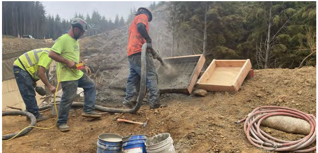
View of contractor applying shotcrete to test panels.
