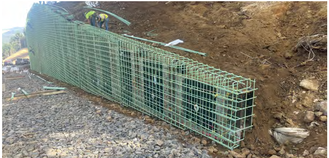
View of soldier pile wall reinforcing bar placement nearing completion.
