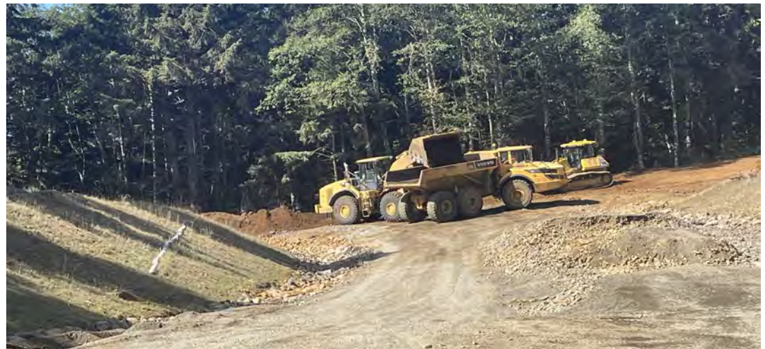
View of existing base aggregate removal near south entry of project.
