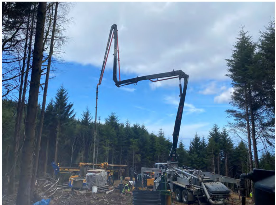
Pouring concrete in the drilled shafts
