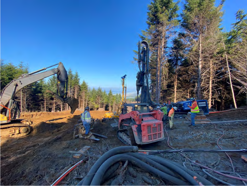
Drilling for ground anchor installation
