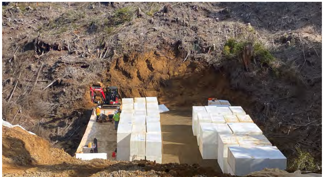
Geofoam wall installation
