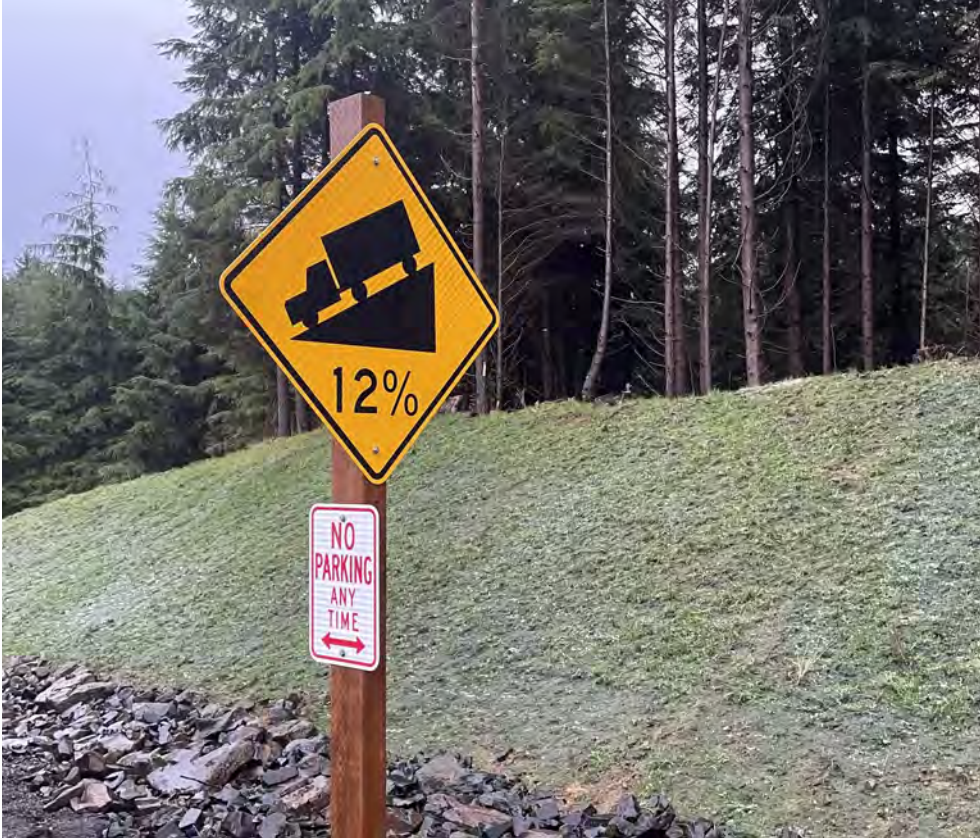
View of newly installed sign warning of steep grade.
