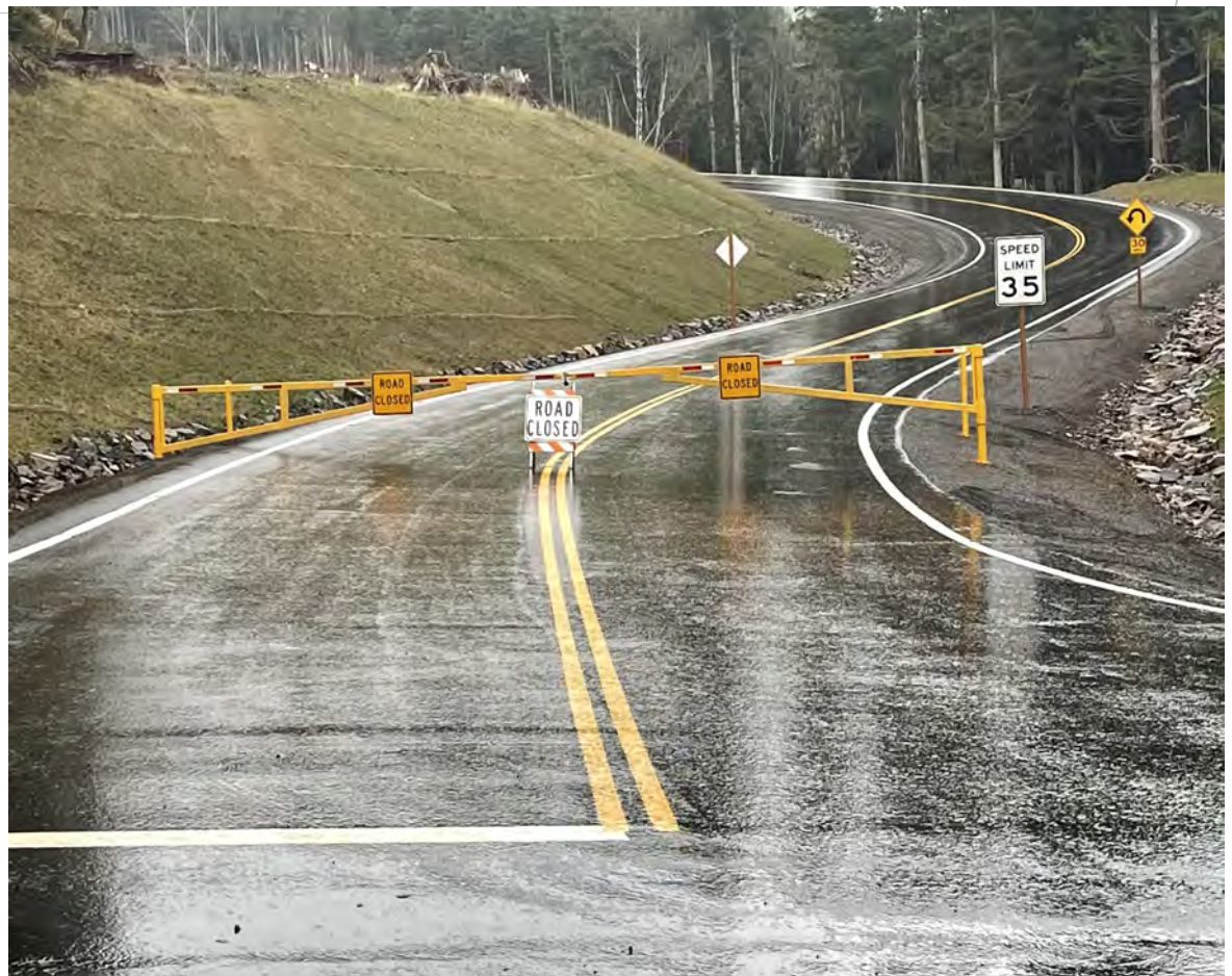
View of South end of project with Tillamook County gates.
