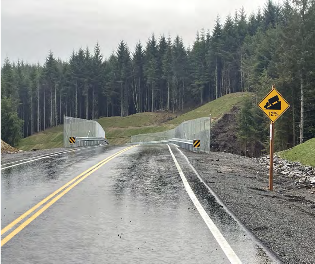
View of Geofoam Bridge at top of northbound 12% grade
