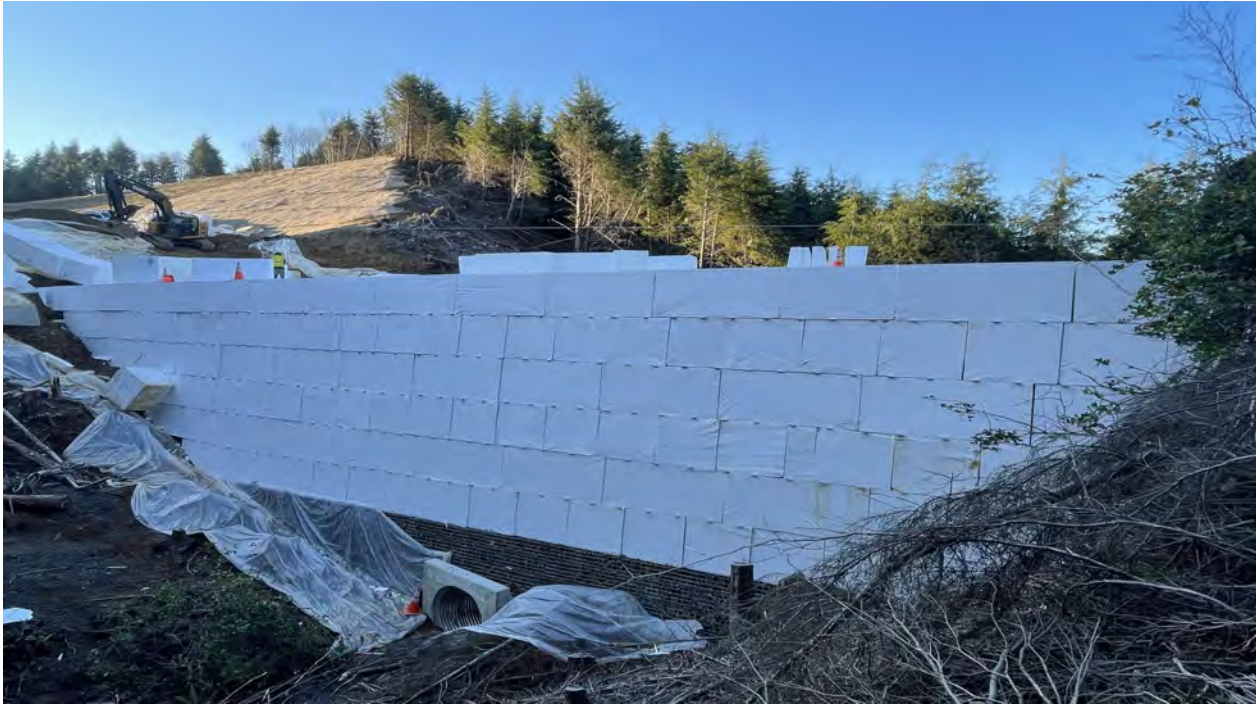
Geofoam wall progress
